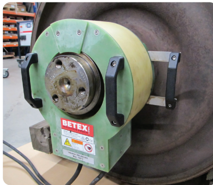
Heating bearing rings for dismounting
